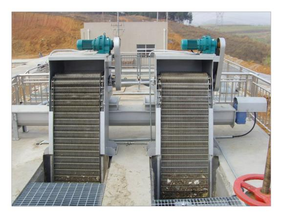
QY series automatic mechanical traveling bar screen is a filter for preliminary treatment, designed to remove debris and other inorganic material from the wastewater to protect downstream treatment process.
